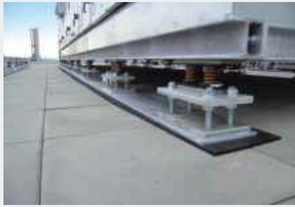
On-roof installation of an HVAC system with relatively high wind loads
