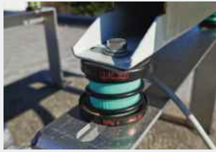
Monoblock heat pump with Isotop DMSN
