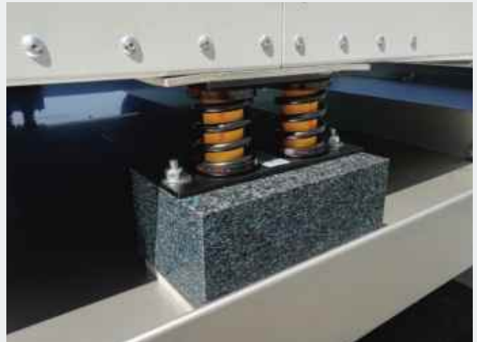
Air conditioning unit with Isotop DT and Isotop DSD-BL2 (not included in the scope of supply)
