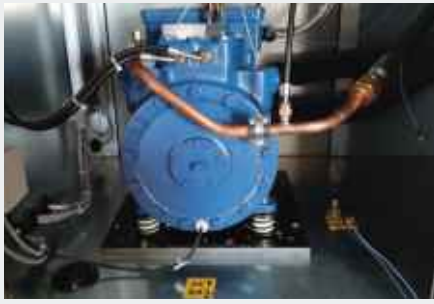
Reciprocating compressor with Isotop DMSN
