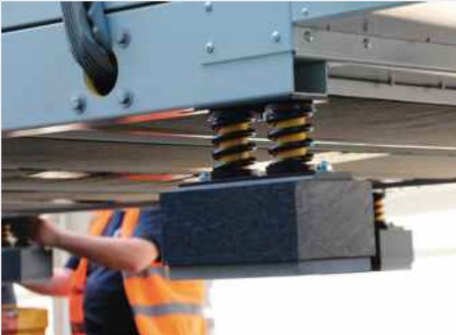
Isotop DT pre-mounted on device frame
