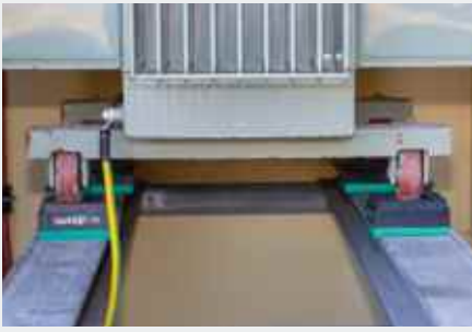
Vibration decoupled bearing of a distribution transformer
