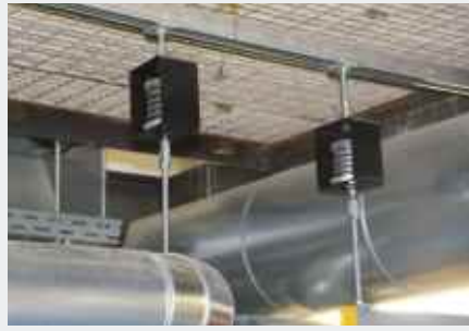
Decoupled pipes with Isotop SD/Z
