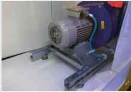
Radial fan in an HVAC system
