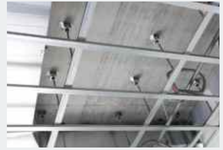
Ceiling hanger Isotop MSN/Z-LC
