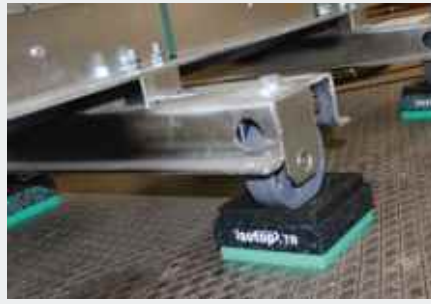
Vibration decoupled bearing of a distribution transformer
