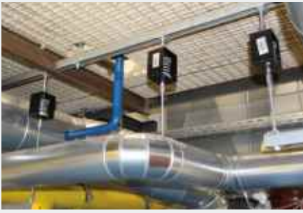
Pipework suspension with Isotop SD/Z
