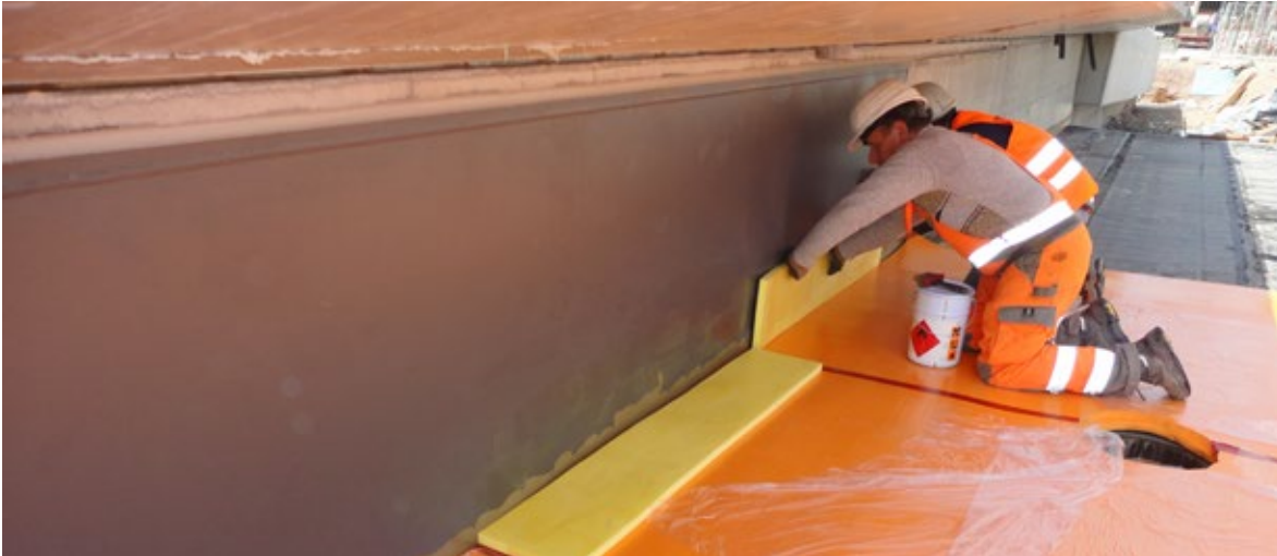
Installation of a mass-spring system
