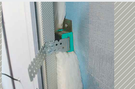
Dry lining decoupled with Sylomer® for high damping efficiency
