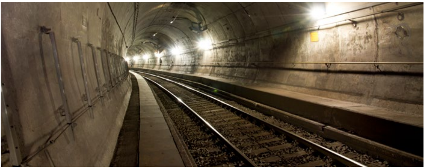
Tunnel Gasteig, Munich
